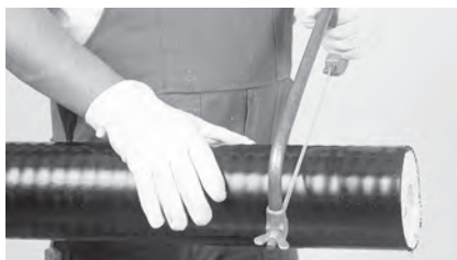
2 Cut the casing pipe with saw.
