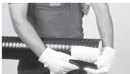
4 Peel off the casing.
