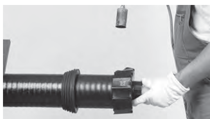
7 Carefully shrink on the pipe end closure according to the Raychem DHEC installation instruction.
