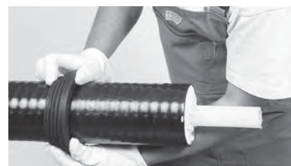
6 Install the wall sealing ring.
