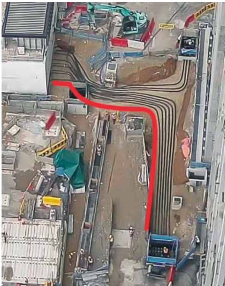
Figure 1: Uninterrupted Pipe Run
